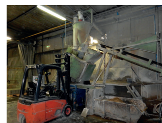
Photo 3, Fork lift truck for internal transport of mixed concrete.
